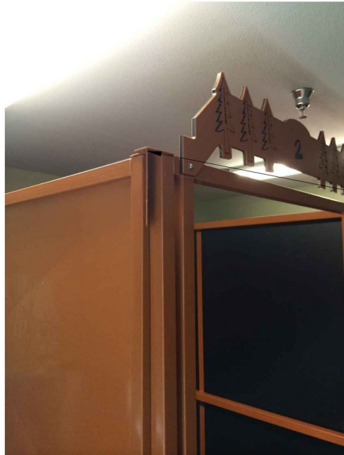
3WAY OR 4WAY CLIP DOES AT TOP AND BOTTOM OF EACH CABIN CONNECTION POINT
